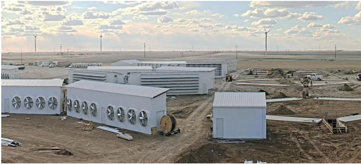
Figure 5. Soluna Data Center Construction at Dorothy
